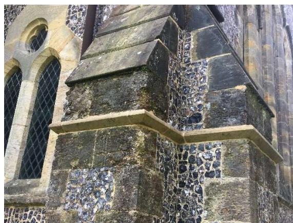
String Course Stonework before and after completion, Spring 2021
